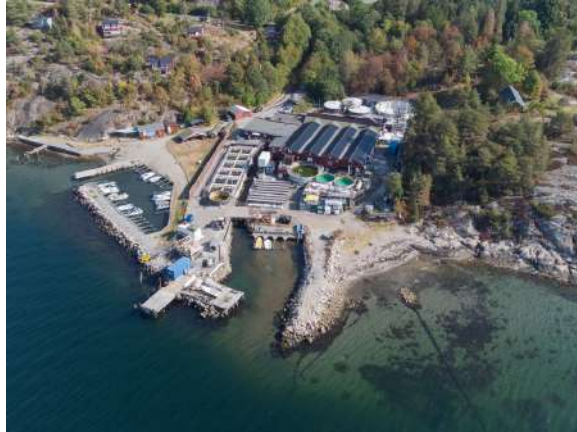
Figure 4. NIVA Solbergstrand Research Station.
