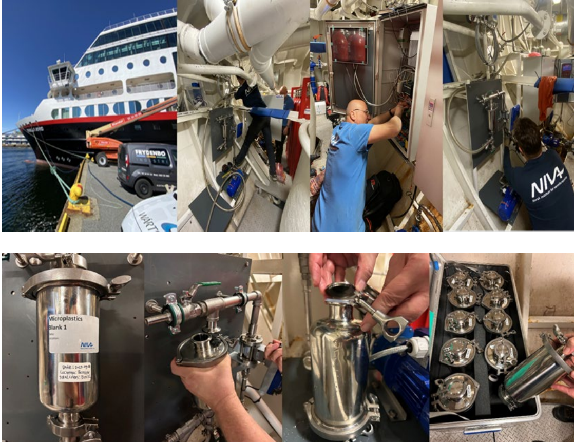
Figure 20: Installation of the microplastic sampler system on the MS Trollfjord.
